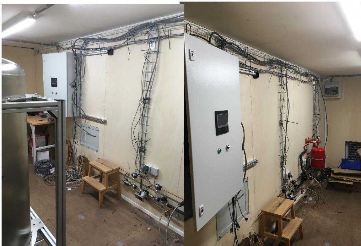
Figure 3: Day 3 of construction.
