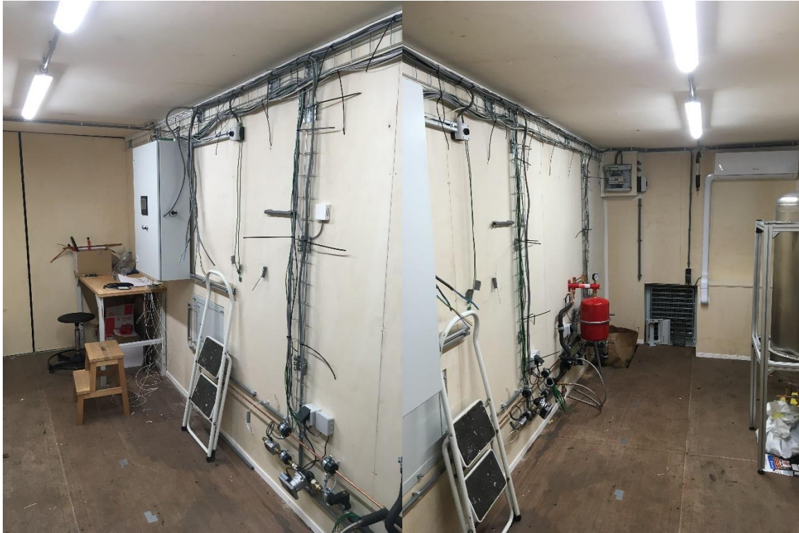
Figure 4: Day 4 of construction.
