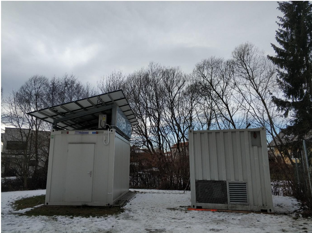
Figure 13: Placement of the CLC Emulator Demo Container to its final location at SCORES DEMO A.
