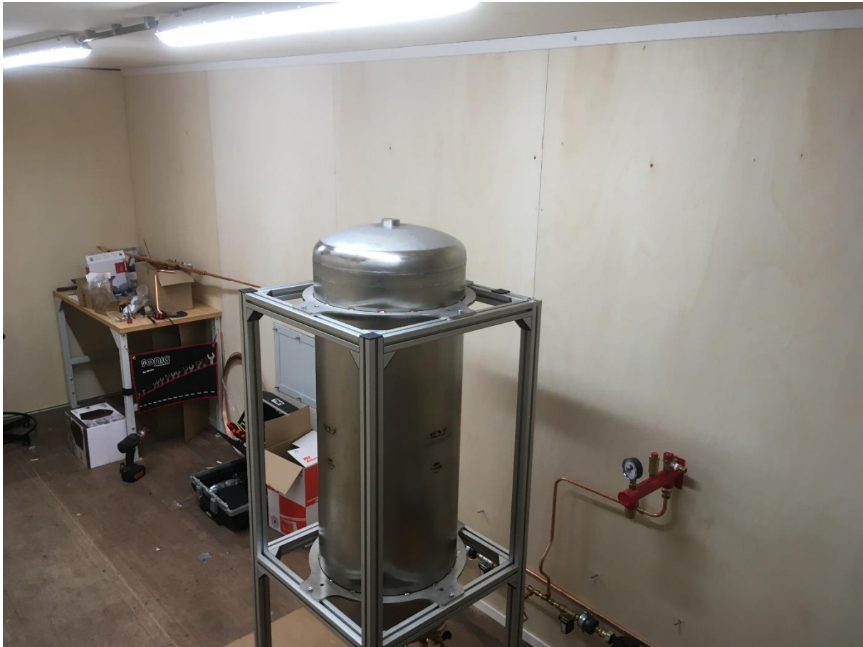
Figure 2: Day 1 of construction.
